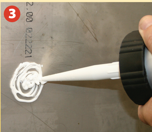
3 Spread a generous layer (2-4mm) of adhesive as shown; make sure the amount you apply will cover the whole head area of the BigHead to be fixed, for maximum strength.
